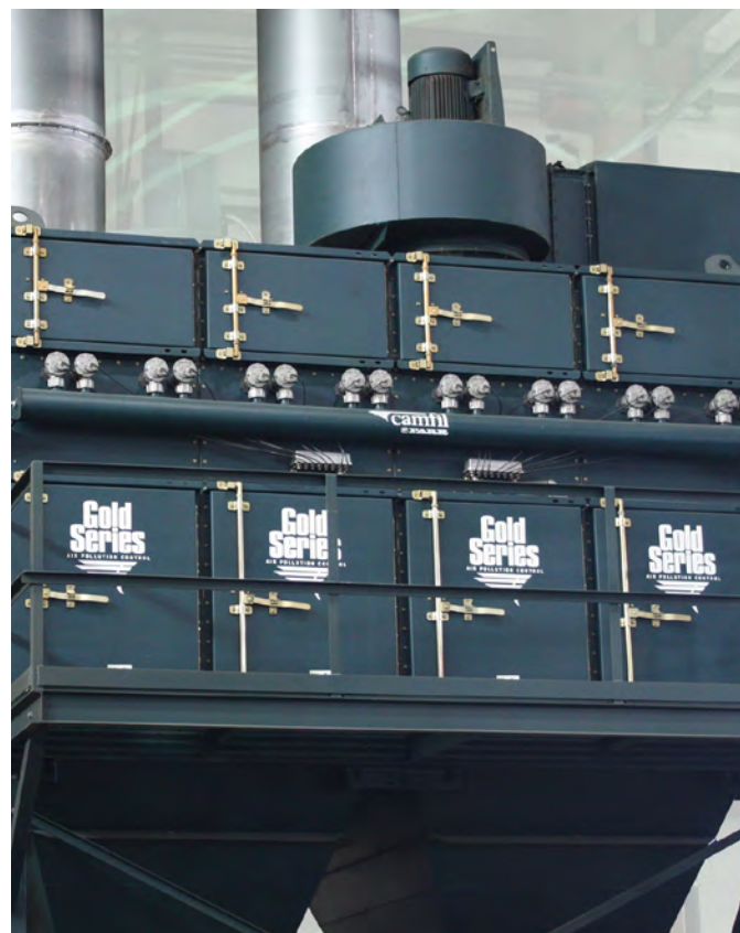
HEPA safety monitoring filters are integrated on top of this dust collector, eliminating the costs of additional ductwork. Mounted downstream of the HEPA filters, the fan is protected against wear and tear from exposure to abrasive silica particles.
